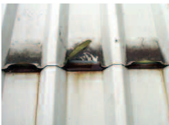
Leathergrain alternative on hot dip galvanised steel substrate roof after 7 years.
